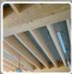
Ceilings and plinth walls
